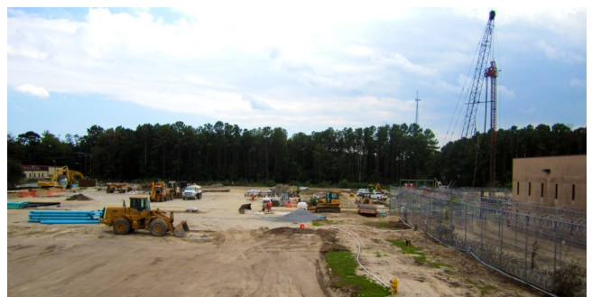
Above: Crews have been using a lot of heavy equipment to prepare the old employee parking lot for the new addition to the Enforcement Bureau.
